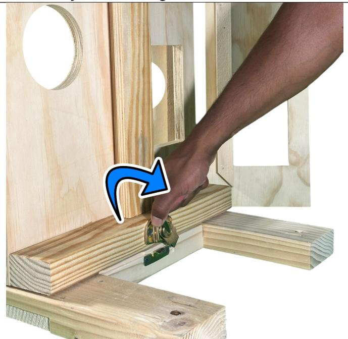
Lock the leg in place by rotating the handle of the sash lock counterclockwise.
